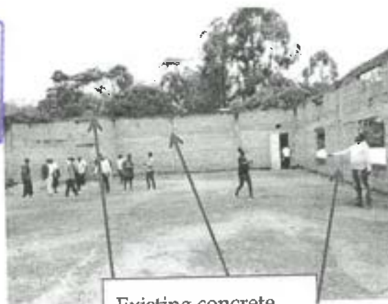
Existing concrete structural elements
