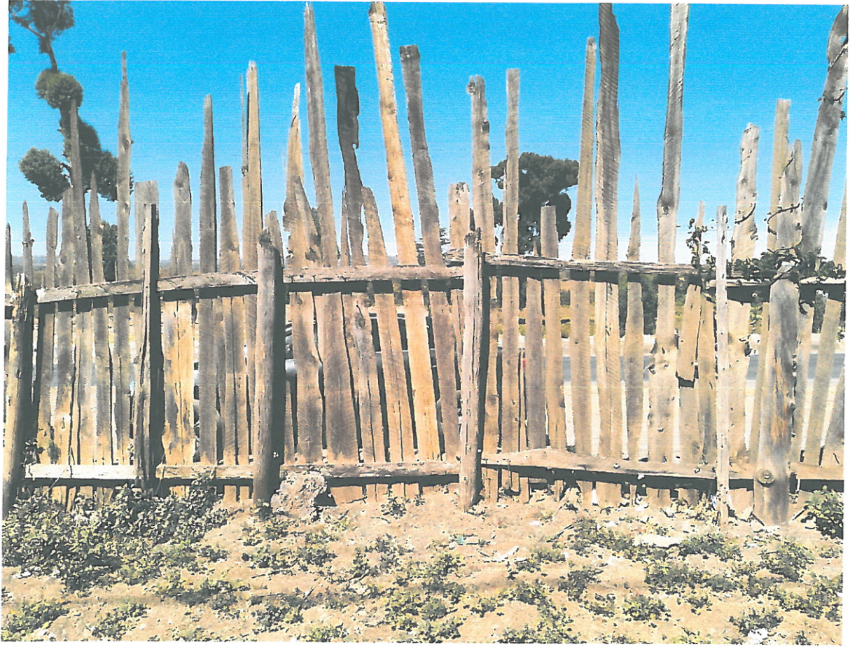
Fence to the Road Frontage
