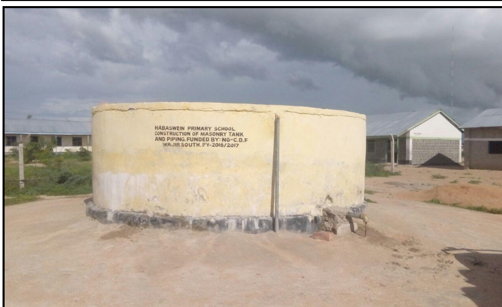
Masonry Tank at Habaswein Primary School
